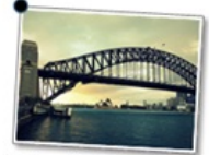
Sydney Harbour Bridge
